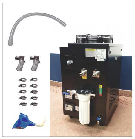
1. Attach the 760-mm inlet hose (P/N: 012-103791-XX) to the chiller **Inlet** port.
