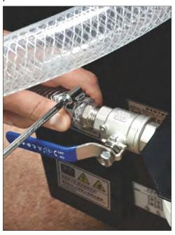
3. Attach the 75-mm outlet hose (P/N: 000-109320-XX) to the chiller **Outlet** port.
