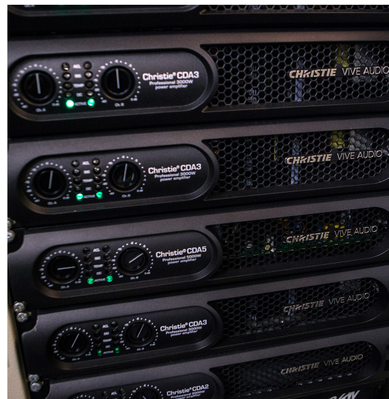
▲ A rack of Christie Vive Audio Class D amplifiers powers the audio system from the projection booth.
