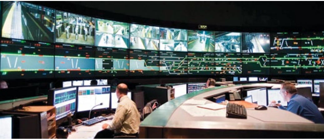
▲ Massachusetts Bay Transportation Authority, Boston, MA
